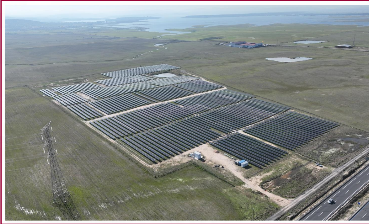
Calzada de Oropesa photovoltaic generation plant in Toledo 7.6 MW capacity 17K modular solar panels
